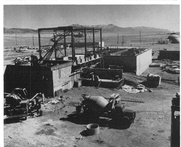
SERF SITE-Most underground construction for Sandia's new Engineering Reactor Facility is nearing completion. Concrete block walls are now being
